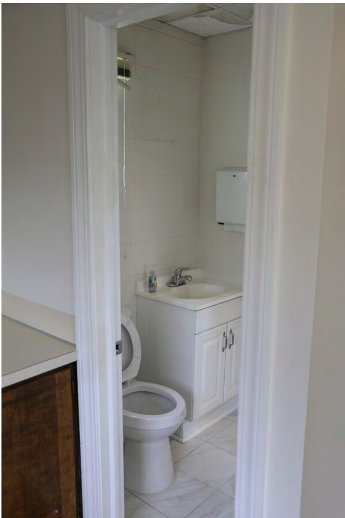
Separate Office Bathroom
