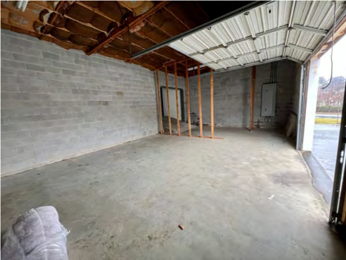
Ground Level Door Area
