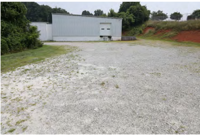
Dock Access Area
